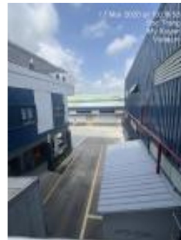
Factory exterior 3.jpeg
