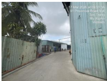
Factory exterior 4.jpeg
